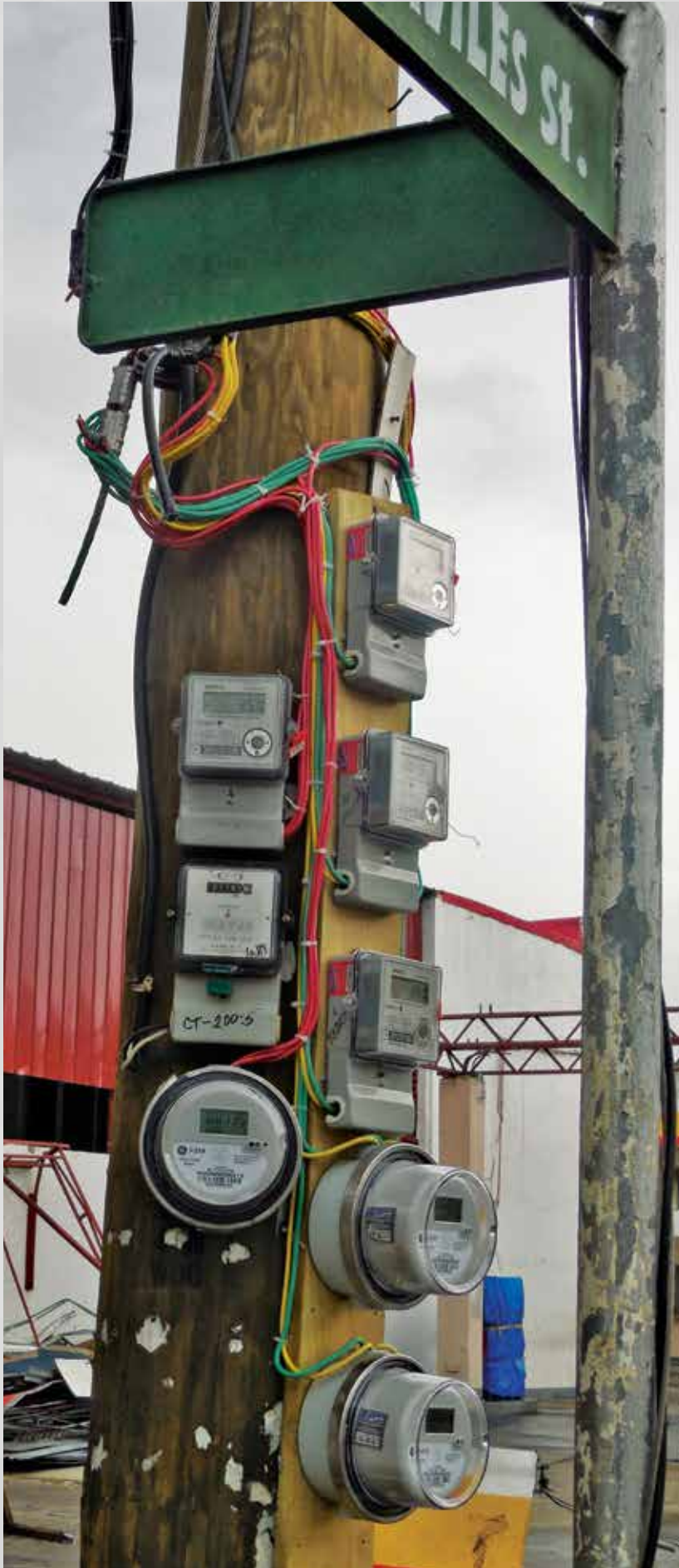
Typical individual meter location
